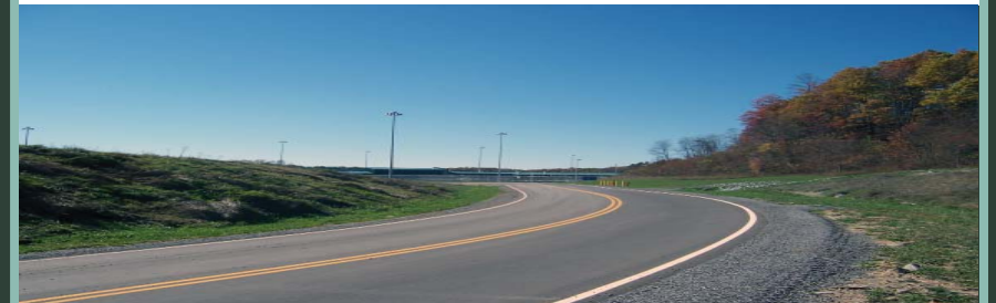
Pocahontas State Correctional Center Access Road Tazewell County, Virginia
