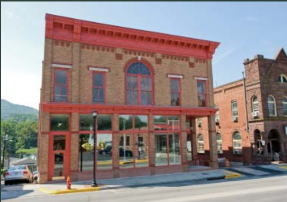
Tazewell County Administration Building Restoration and Adaptive Reuse Tazewell, Virginia
