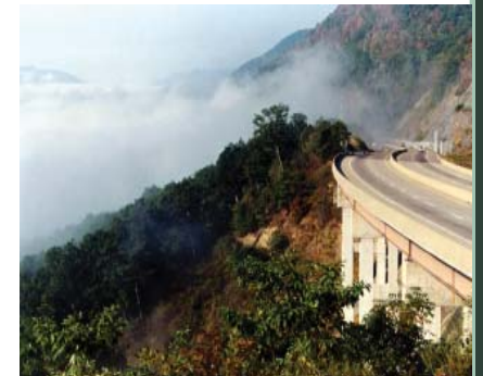
Powell Valley Bridge
